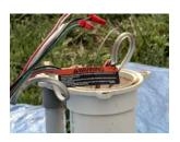
▶ If your well has a well cap, remove the bolts along the outside edge of the top of the well cap for newer models, or loosen the set screws on the side of the cap for older models and lift off the cap. Gently lift the wires/wire nuts out and pull to the side. Do not pull on the release cable or pull the pipe for the pitless adapter and pump. Check for damaged wires/wire nuts. Be careful not to loosen any connections.
